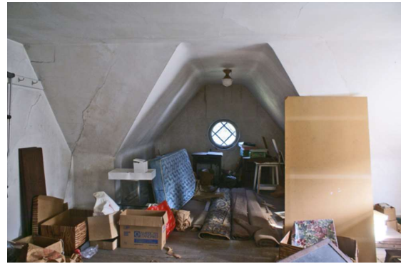
Plastered Attic Southern Addition
