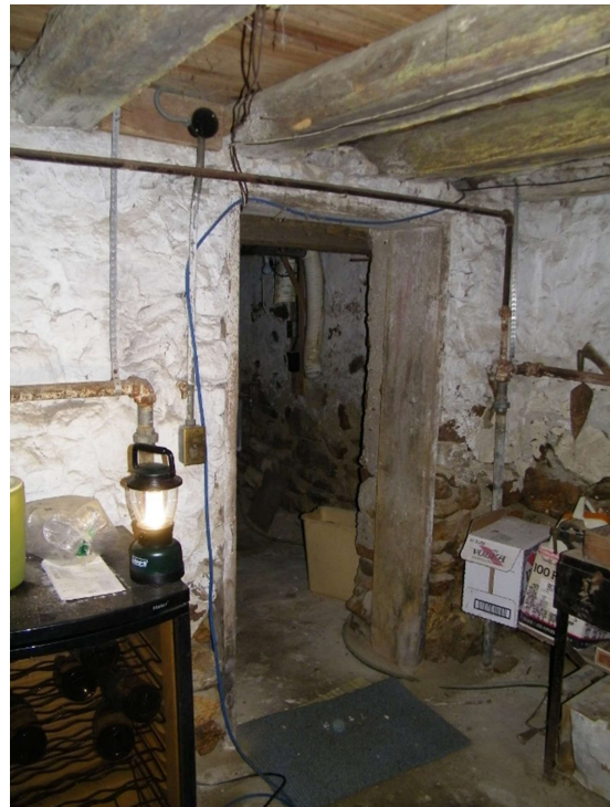
The original basement had log ceiling joists.
